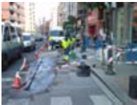
Figure 2 Delivery space roadside installations
